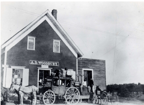
The Woodbury Store and Post Office
