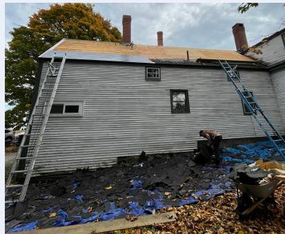
Work Begins On The New Roof
