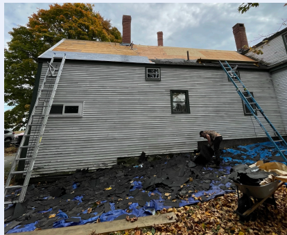
Work Begins On The New Roof
