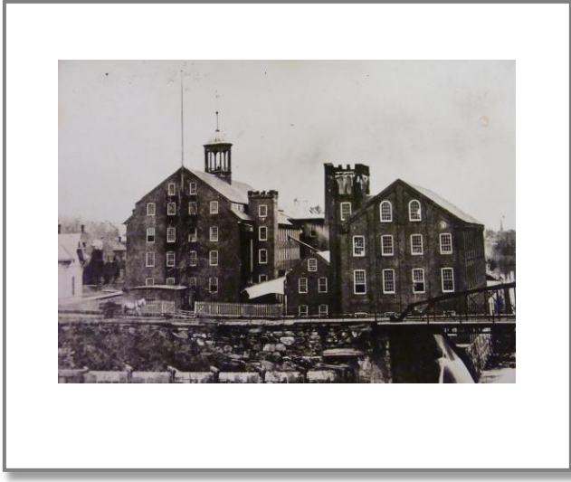
Mills and dam – Bridge Street bridge
