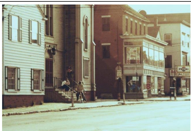
Figure 2 Main Street at Brackett Street
